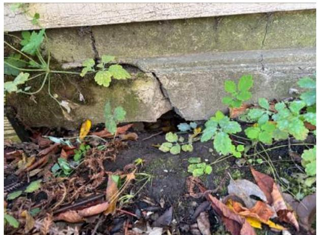
**5. Interior Slab and Foundation/Structure Settlement**
