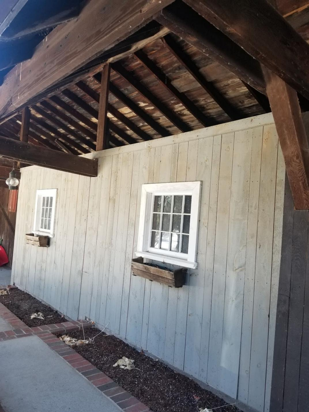
This is the exterior wall that will remain: it will be built up to the rafters and the window on the left will be replaced with a door.
