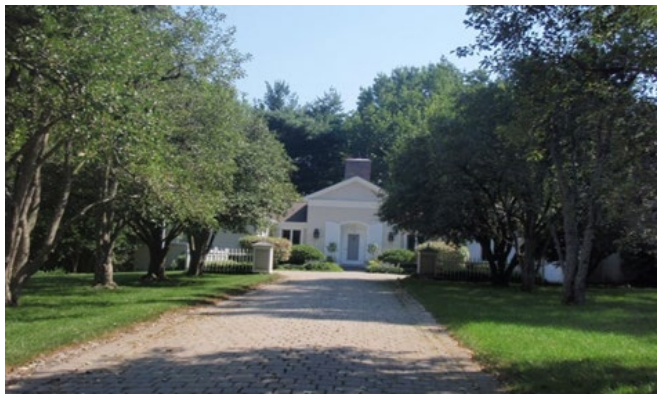
The formal "entry court" on this house provides an attractive entry while screening the garage and parking area from the street.
