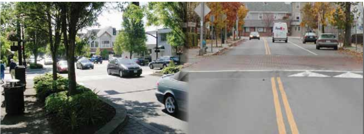
Traffic calming in action. Left: bulb outs, raised median, and textured crosswalk in Oregon. Right: speed table with crosswalk in New Jersey.
