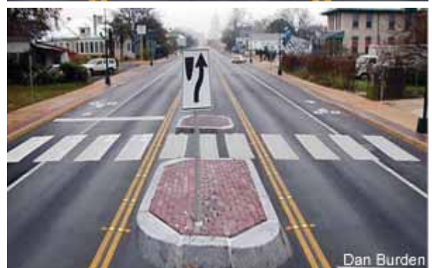
Road Diet. Top: Original road. Middle: After road diet – four lanes become three lanes plus bicycle lanes. Bottom: mid-block pedestrian crossing island added in the center lane.
