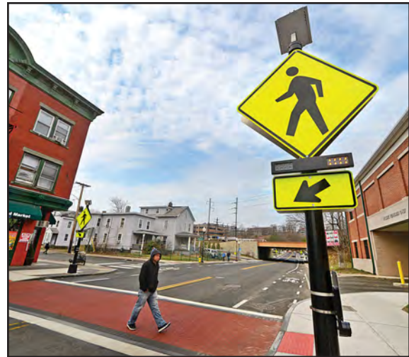
Rectangular Rapid Flash Beacon. Photo by The Hour.
