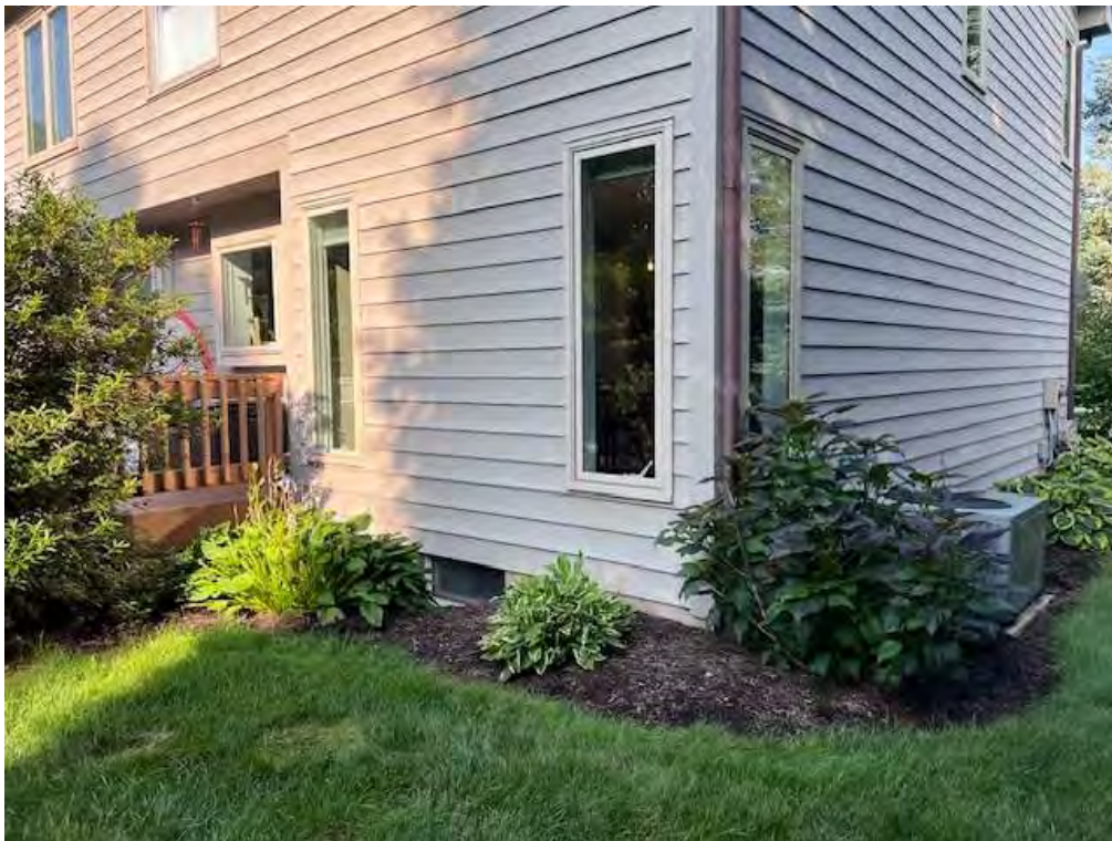
Rear of 20 Meadow Cove Road (Windows making for difficult placement)
