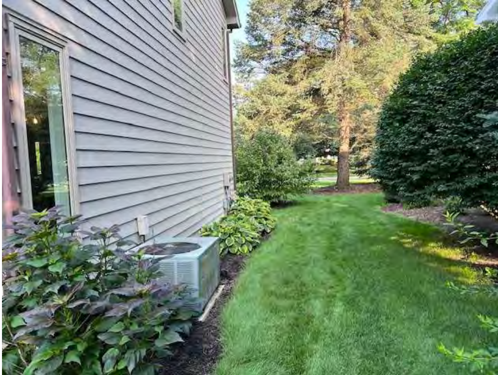
Proposed location of the equipment (Between 18 and 20 Meadow Cove Road, 14534)
