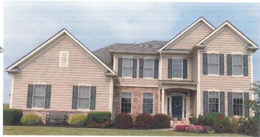
Existing House @ 5 Pepperwood Lane
