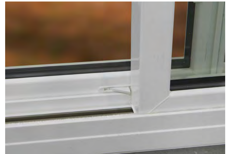
Push button spring-loaded vent latches allow both window sashes to remain partially open for ventilation.
