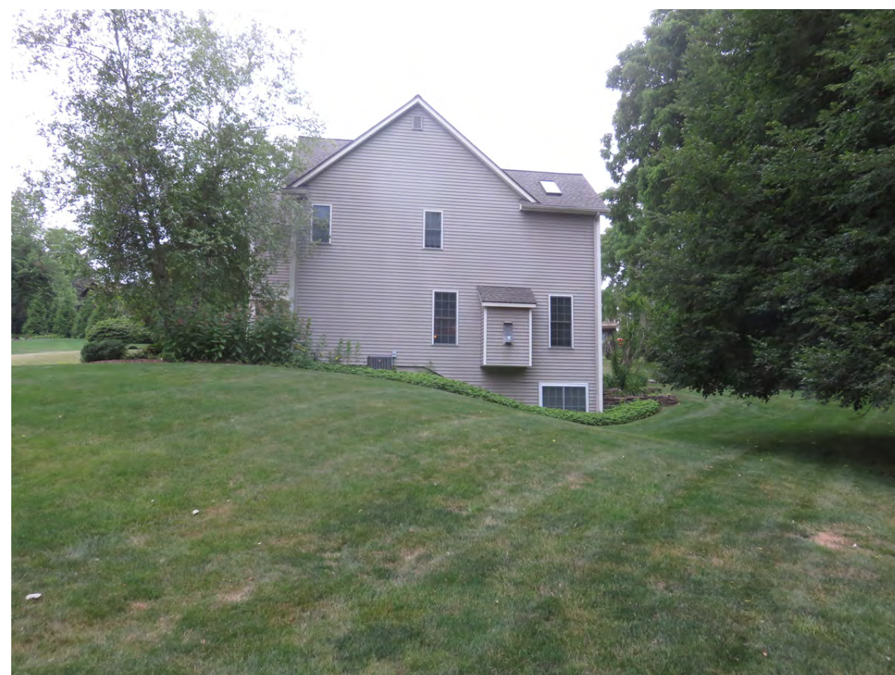
EAST ELEVATION. (from Mill Rd)
