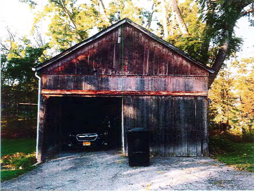
682 Stone Road - Goldman Residence Existing Garage - 10.12.2021
