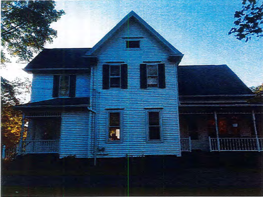
682 Stone Road - Goldman Residence Existing House - 10.12.2021
