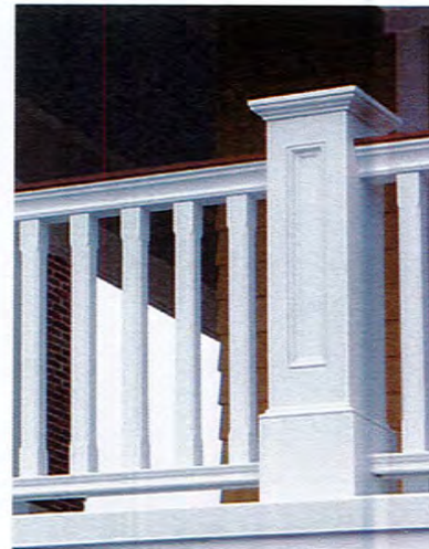
PORCH RAILING: EXISTING TO BE RESTORED AND REPAINTED. NEW RAILINGS TO MATCH EXISTING
