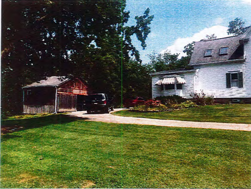
682 Stone Road - Goldman Residence Existing Barn, House & Garage - 10.12.2021
