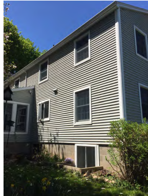
South-East Corner of House
