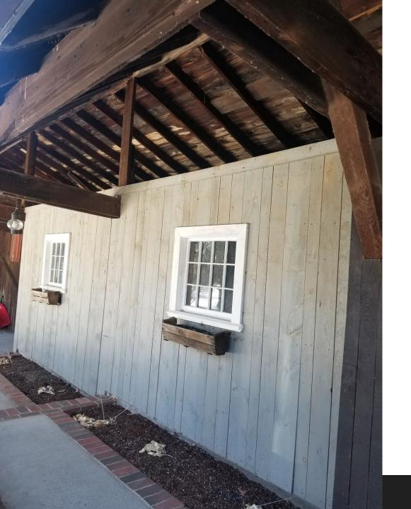
This is the exterior wall that will remain: it will be built up to the rafters and the window on the left will be replaced with a door.
