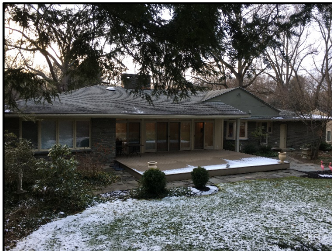
Rear View with Patio and Deck, January 2021
